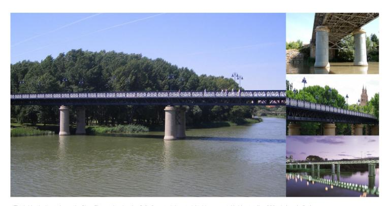
The bridge is situated over the River Ebro prolonging the Calle Sagasta. It is a straight 11 span metal bridge totaling 330m in length. Both abutments are made of sandstone masonry.
